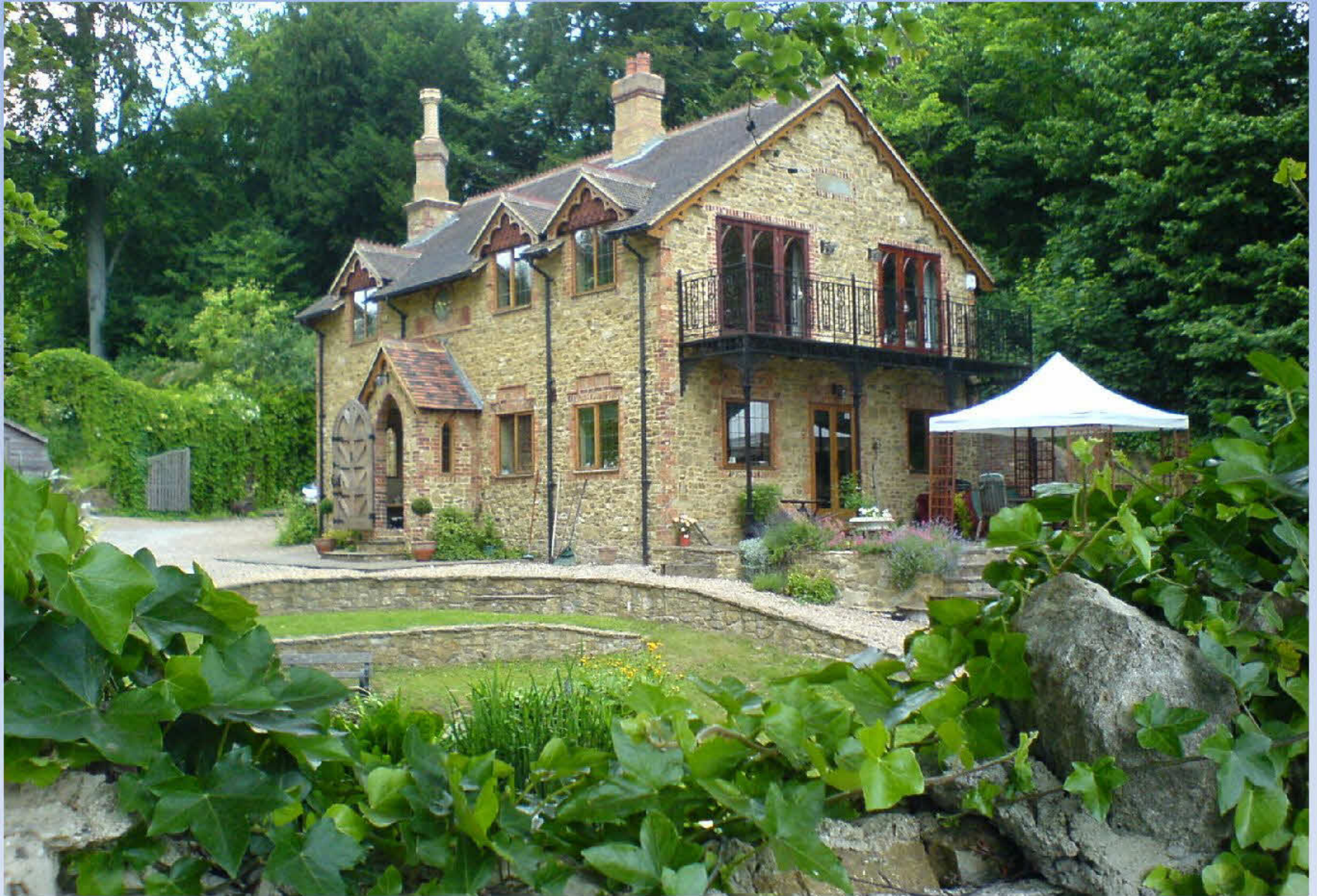
Weycliffe House Portsmouth Road
